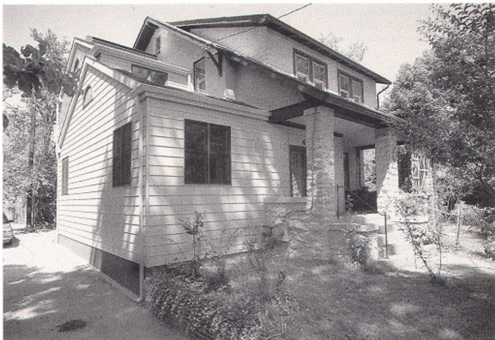
Exterior appearance as well as interior space was carefully considered when this room addition to a Washington, D.C., home was planned. Aluminum siding that closely matched the existing stucco made it unnecessary to re-paint the original house. The siding was extended midway across the front porch to tie in the addition.
