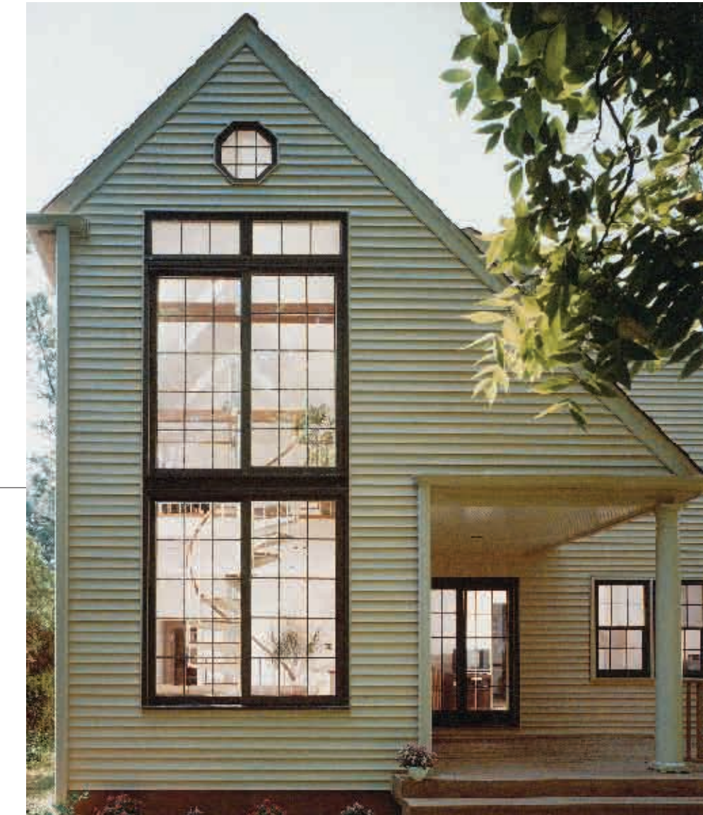
ABOVE: The new rear addition creates a sheltered entrance to the garden. Photograph by Daniel Peck Photography
